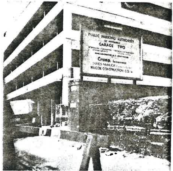
PARKING AUTHORITY RAMP GARAGE - PROJECT No. 2 Pittsburgh
