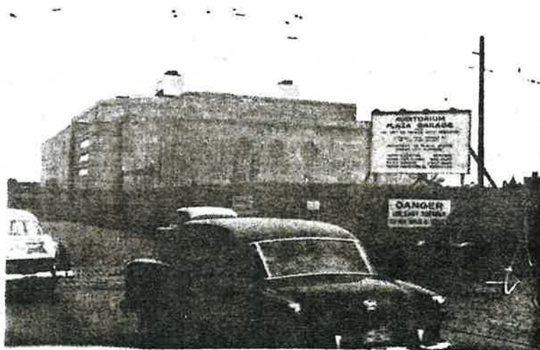
Municipal underground garage under construction
