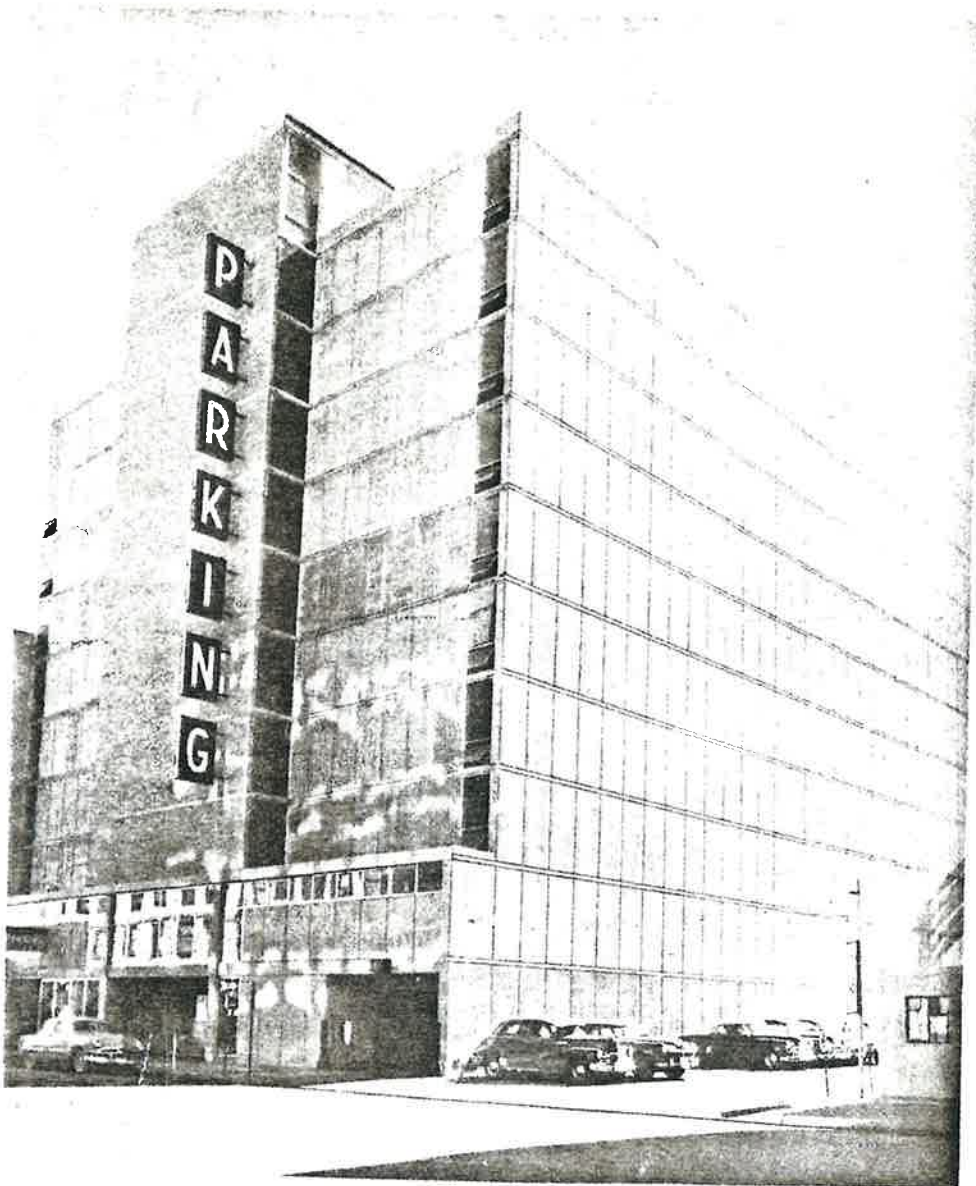
ONE OF THREE MUNICIPAL GARAGES Bowser Mechanical Design
