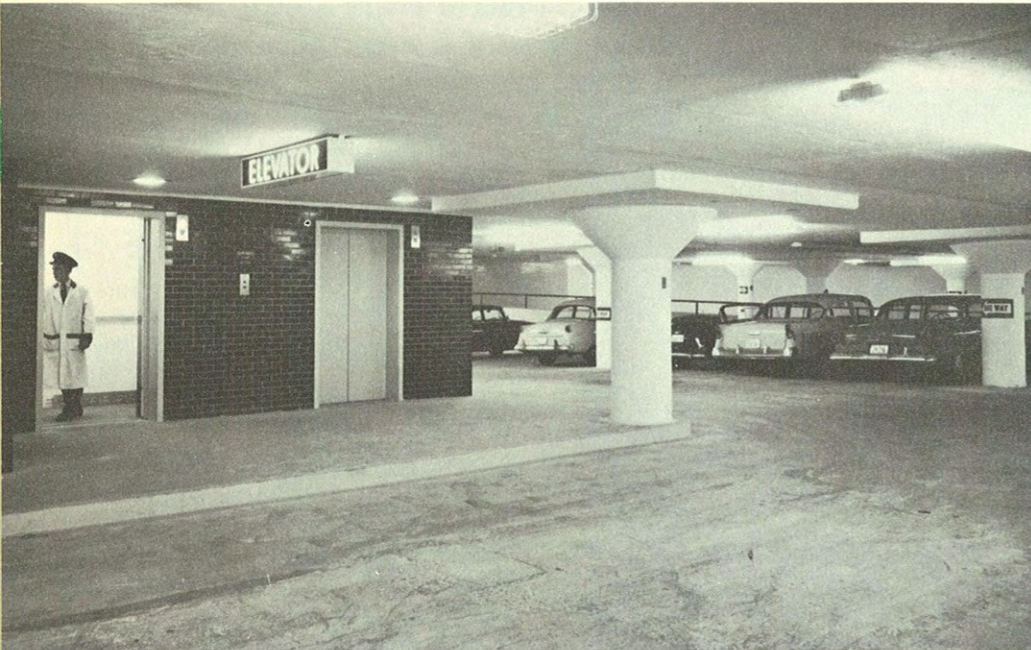
For the convenience of motorists, the underground garage is serviced by passenger elevators from all floors to the surface.
