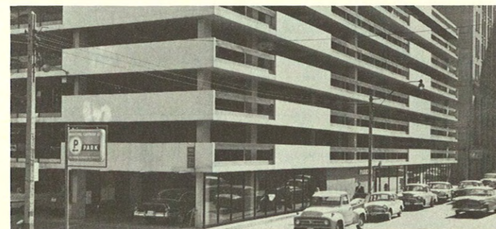
Mechanical Garage Temperance Street
