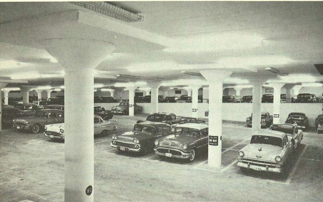
A view of the interior of the underground Civic Garage, showing adequate lock-up facilities and turning space for each vehicle.
