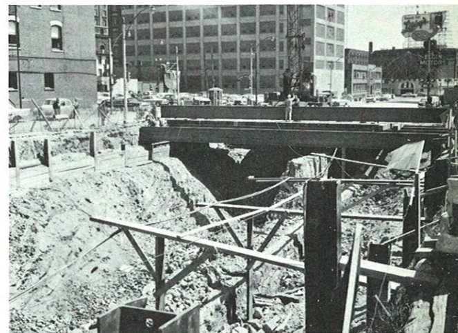
Decking Operation north of Wellington Street
