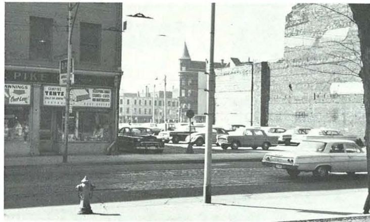
Extension to carpark No. 14.
