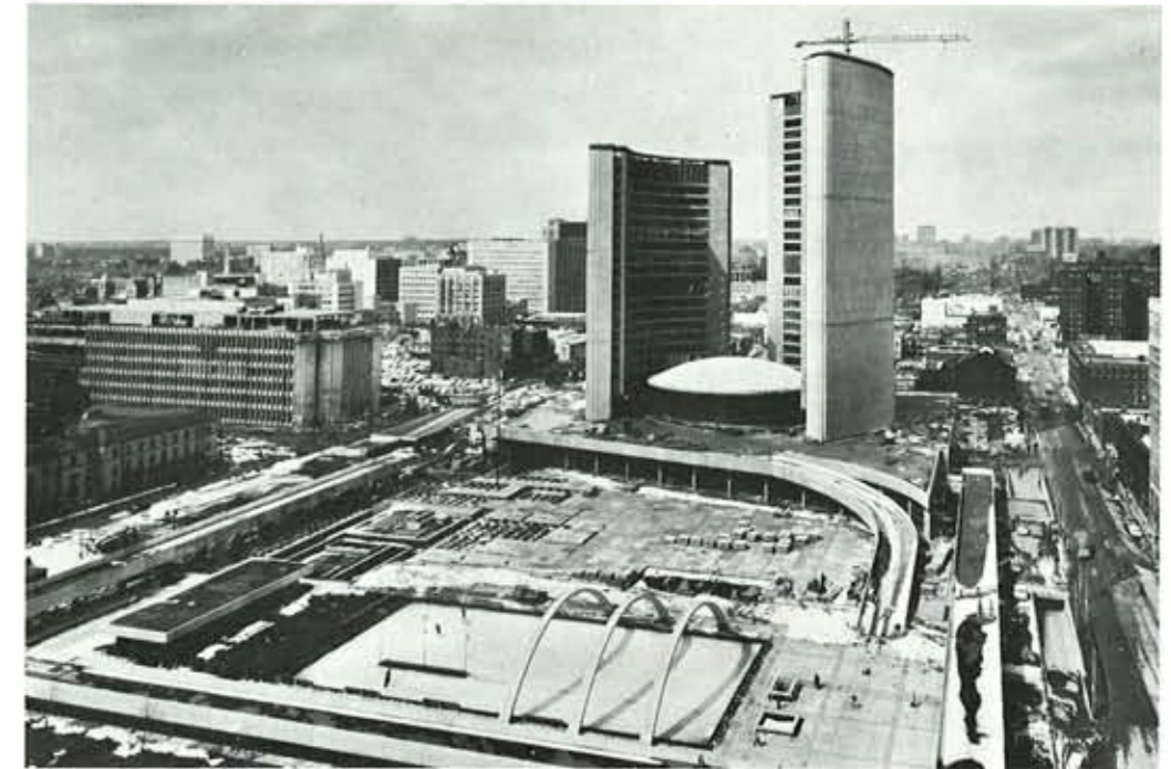
Underground Parking Garage Nathan Phillips Square
