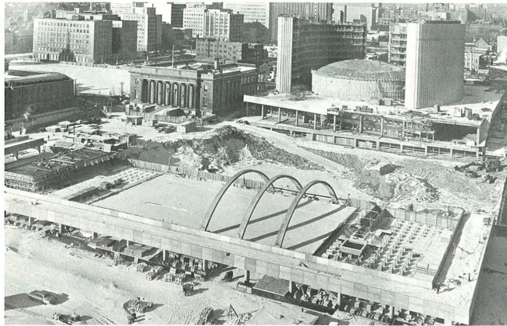
Underground Parking Garage Nathan Phillips Square
