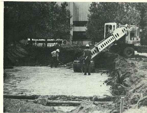
Removal of landscaping above Queen St. entrance
