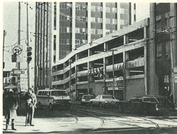
Municipal Carpark 26, south side Queen Street E., at Victoria St.
