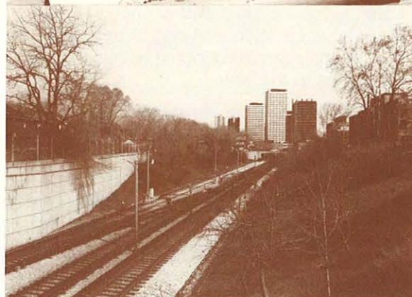
Open-cut subway line in the Yonge-Davisville area
