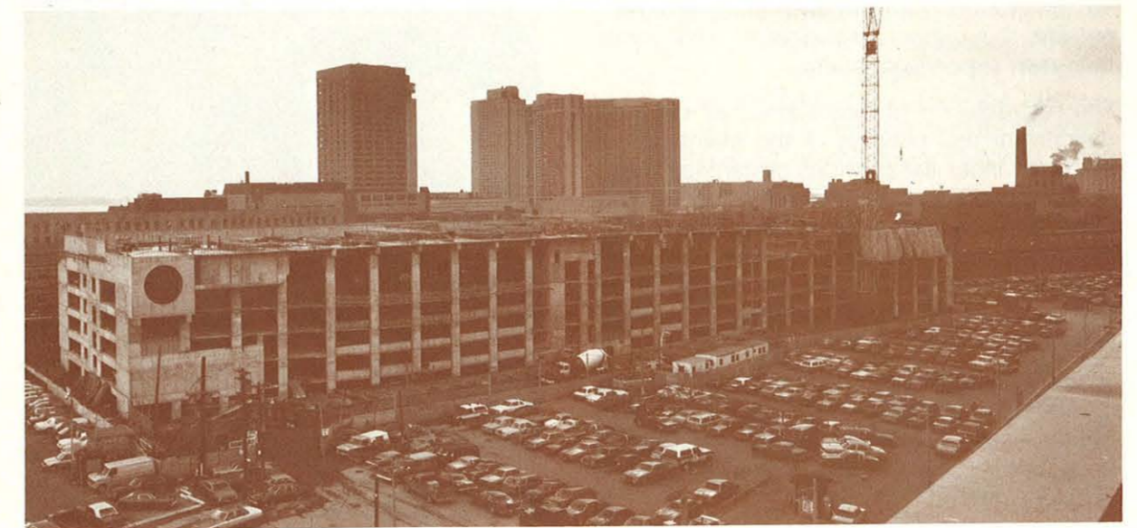
Municipal carpark 43, the St. Lawrence Garage under construction.
