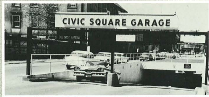
Entrance and exit at Queen Street West for the garage under Nathan Phillips Square, built in 1958.
