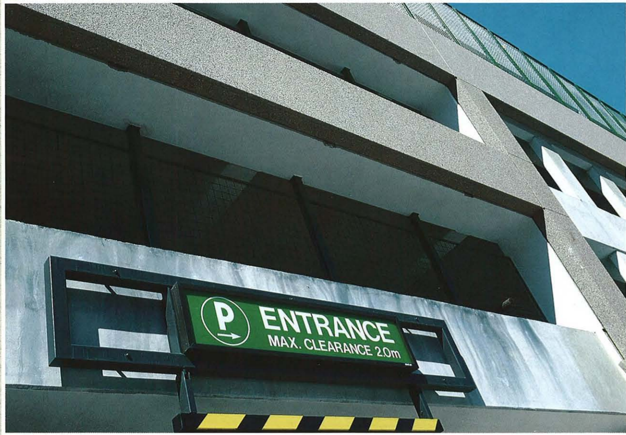
The Queen/Victoria garage was designed to be both operationally functional and architecturally attractive. The result is a municipal parking garage which enhances the streetscape along Queen and Richmond Streets.
