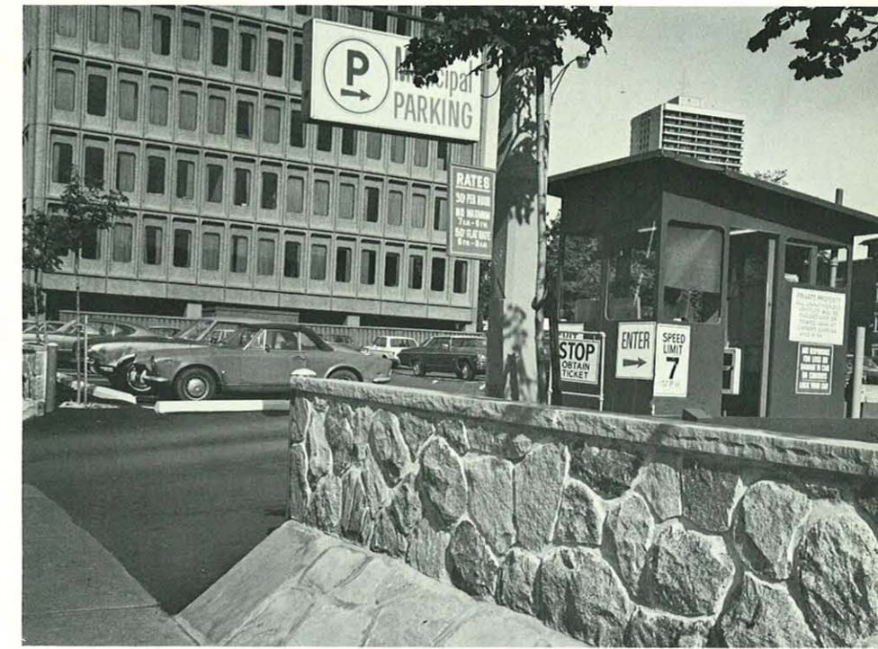
Off-street carparks are made as attractive as possible to complement the surrounding area.
