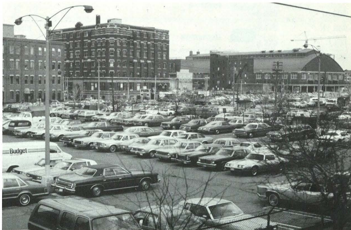
Carpark 43 before construction
