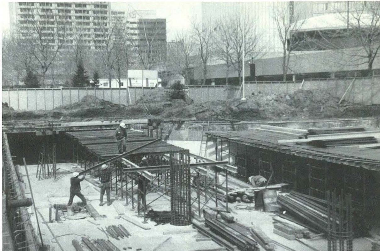
Reconstruction of the Queen St. ramp, Carpark 36
