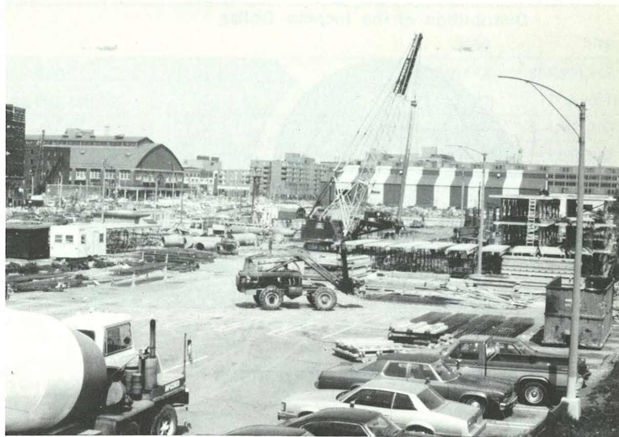
Construction of Phase C-1 St. Lawrence Garage on Carpark 43
