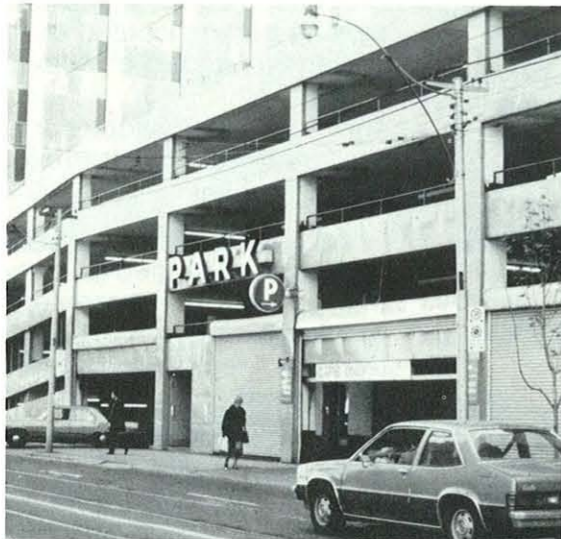
Carpark 26, Queen St. - Victoria St., soon to be rebuilt
