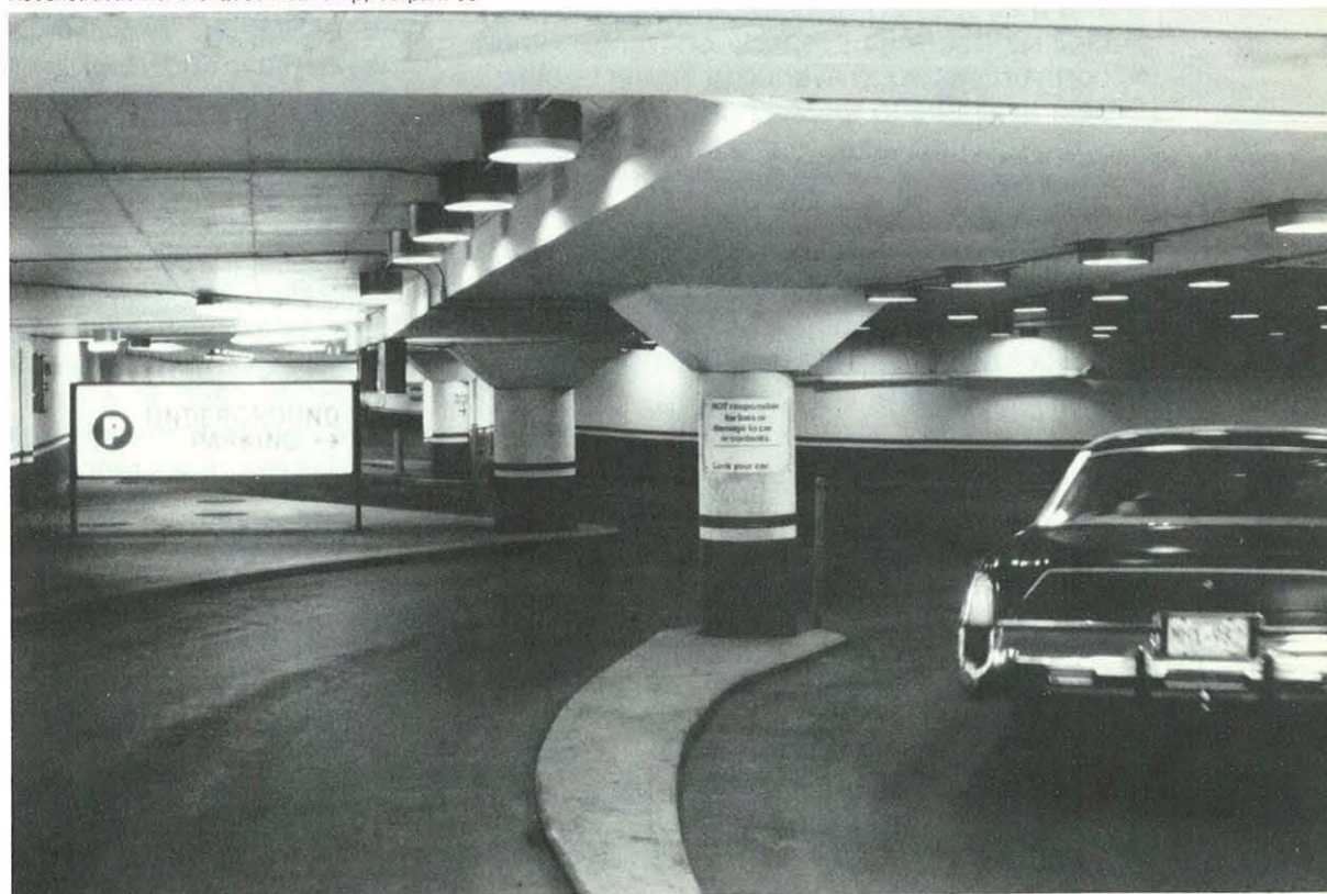
Completed ramp, Carpark 36
