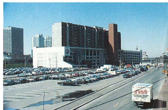
Careful planning includes provision for future expansion. The eastern wall of the St. Lawrence garage shows sections of knockout panels that can be easily removed to connect all floors of the present garage with a future 850 space extension.
