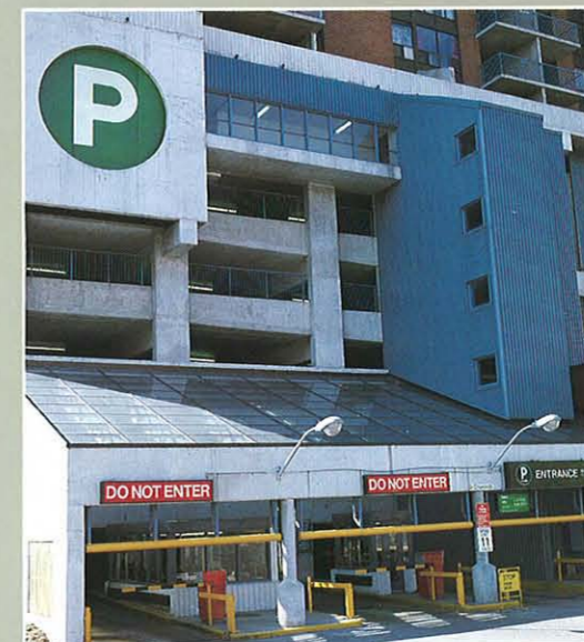
The Authority has accelerated plans to expand the St. Lawrence garage, its second largest facility, by building a 950-space extension at that location.
